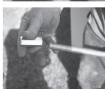
**8.** Attach a connector nut to the threaded rods and then attach the 6" inch stainless steel threaded section to the top of the connector nut.
