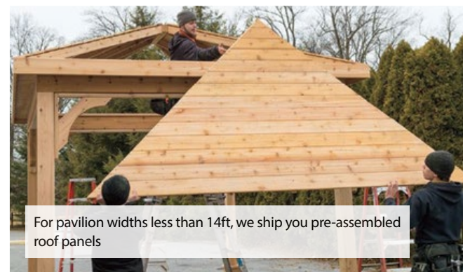
A) We notch the tops of your 6x6 posts 1 1/2" on both sides to fit your 2x8 beams, and B) we notch your 2x8 beams 1 1/2" deep to fit your 2x6 rafters
