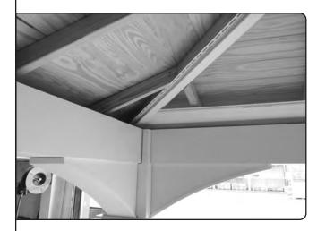
**3.** Install first piece of ceiling panel, placing 1" nails on each rafter.
