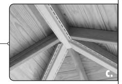
**2.** Install T-channel on hip rafters. Push down into lower gap against plate (a), the mark and cut top to fit. (b, c)
