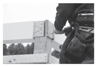
10. Once you have the two long side headers up, put the shorter ones on. These get fastened to other headers with three 3½" screws. Use the three predrilled holes going into other header.
