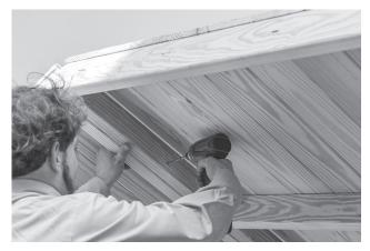
35. Fasten the ridgepole together with one  $2\frac{1}{2}$ " screw every 16". Use step 34 and 35 with other two panels.
