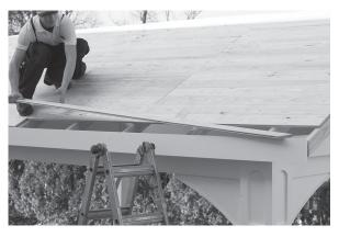
43. Now you are ready to fasten rafters to plate. You have to remove bottom pieces of 1x6 T&G board. It will be screwed on. Just back the screw out and remove the board.
