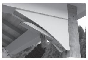
21. Once you have all the braces installed, put the 2x4 block back in place. Fasten with two 2½" screws.
