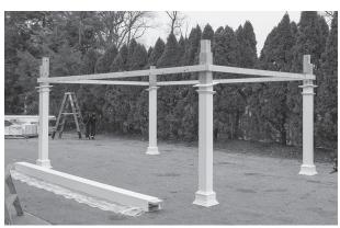
8. When you have all posts at marks, get the template and fasten it to tops of post. Make sure all post components are on. As you cannot put these on later. Make sure all posts are level and everything is square.
