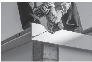
14. Next step is installing the fascia boards. Install the two shorter ones first. These go up past the plate about 1%" for asphalt shingles and 1%" for metal roof. Fasten with one 2%" white head screw every 16".
