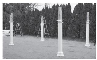
7. If you ordered an electrical package, there will be a 6x6 post with a notch in one side. Put the sleeve with receptacle on that post. Make sure all posts are at the marks you made with template. That would be the inside core of 6x6 post.
