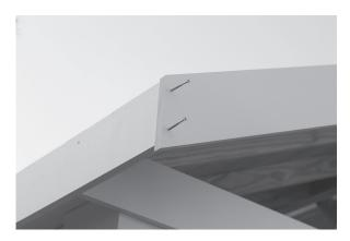
42. Fasten the bottom with two screws going into long side fascia. Continue with rest of pieces.
