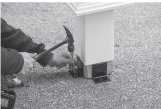
27. Putting the wedge anchor in, make sure the nut and washer are on. You might need to tap it in with a hammer. When you have it down against the washer, tighten the nut with a wrench. Slide the post base down. Do that with all eight brackets.
