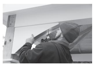
20. Keep the brace flush on the outside of post. Fasten to post with two 3%" screws and up into header with two 3%" screws. Line the brace up with the seam on bottom of header. Do that with all eight braces.
