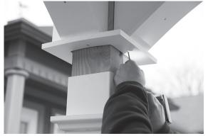
24. Fasten the trim ring to bottom of braces with two 2½" screws.
