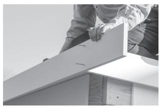
16. Fasten fascia board to gable side fascia with two 2%" screws. Then every 16" with one 2%" screw.
