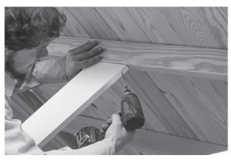
39. Now put the left and right side in. Fasten with one 2½" whitehead screw at the top and one in bottom.
