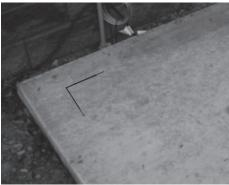
5. Once the template is "square", mark the post locations (using the INSIDE corners of the framed box) on the concrete slab with a pencil. After you have all the post locations marked on the concrete slab, remove and set the wooden template aside.
