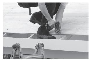
44. When you have all the boards off, fasten each rafter with three 2½" screws. One on each side of rafter toe screwed and one down the center on top.
