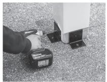
25. Next step, fasten black L shaped brackets to bottom of 6x6 wood post. Slide the 6x6 wood post. Slide the 6x6 sleeve up so the bracket fits underneath it. You can fasten sleeve to post if you want to. It will all get covered. Fasten bracket to post with five 2½" screws.
