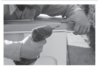
13. Fasten the 2x8 plate to 2x12 plate with one 3½" screw at the corner. Then down into post with two 3½" screws. When you have all four plates in place, put two 3½" screws every 16" plate down into header.
