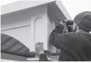
31. Installing the outside corner trim. These will have six predrilled holes. Using the cortex screws, put plugs in. Same as step 30. There will be a tube of caulk in hardware box. You can use it to fill all the seams and cracks.
