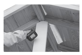
38. Put the longest piece in first. Goes right underneath the rafters and ridgepole right inside fascia. Fasten with two whitehead screws on top and two at the bottom. You might have to cut these if needed.
