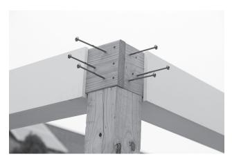
11. Making sure everything is still square and level, install the long 8" GRK screws. 6 pcs. per corner using the predrilled holes.
