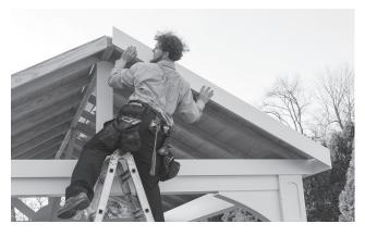
41. Installing the gable end fascia. You might need to cut these to length. Keep it flush on top of roof panel and in center of ridgepole. Fasten with one 2½" whitehead screw.
