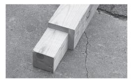
**Note:** The posts are notched on two sides. Turn the notches toward the outside of building.
