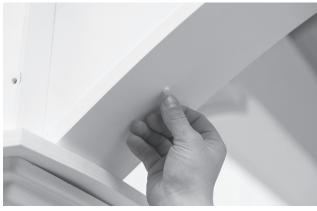
30. Fill all the cortex screw holes with plugs. Tap them in with a hammer until they are flush with trim.
