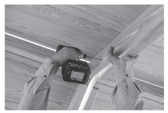
36. Fasten center rafters together with one 2½" screw every 16". Make sure the ridgepole doesn't sag in the center. You might have to put the prop in if it does.
