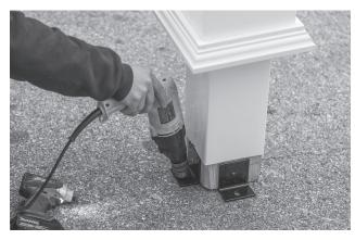
26. Make sure all posts are level and at the marks. Drill down with 1/2" masonry bit about 1/2" deeper than length of anchor bolt.
