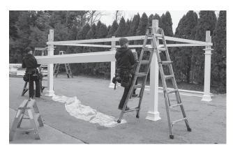
9. Now you are ready to install the headers. Start with the long side. If you have a square pavilion, it would be the shorter headers. It might take three or four guys for this step. Fasten header to post with two 3½" screws. Do not use the predrilled holes
