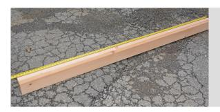
Measure the post, then measure the same height on installation wall and mark it off.
