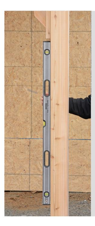
Level the posts on both sides. Fasten the black plates to the posts with 5 2.5" screws catty-corner on the posts as shown.
