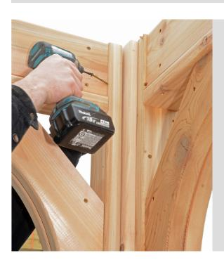
Resten header beam to post with 5 2.5" screws. Make sure header beam is flush on top of post.
