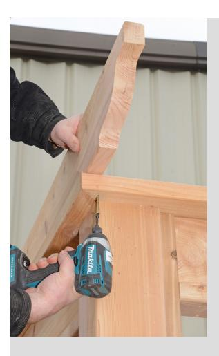
16 Place them on top of plates – align with pencil marks, fasten with 1 2.5" screw on front and back of pergola. Once all runners are in place, add 1 more 2.5" screw per runner on inside of header. (Not pictured)
