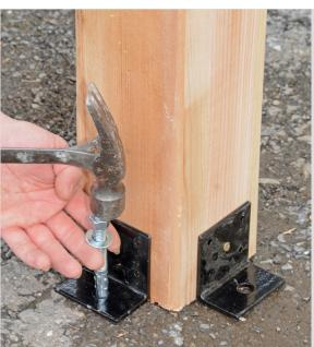
Before inserting the bolt, make sure you have the nut and washer on (otherwise you may hit the bolt too deep into the hole.) Insert the wedge anchor bolts into the holes, leaving about 1/8" of bolt exposed above the nut. (You may need to use a hammer to tap the wedge anchor bolts into the holes.)
