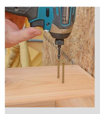
Evenly space the overhangs. Fasten to the header beam with 2 2.5" screws. Fasten top ledger plate with 2 2.5" screws every 16 inches. Finish fastening plates to beams with 2 2.5" screws every 16 inches.
