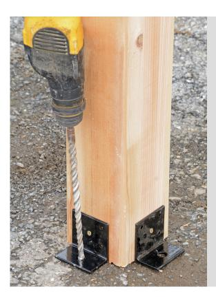
Use masonry drill, drill appx. 5" deep.
