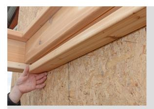
Fasten bottom ledger plate to ledger and mounting with 2.5" screws every 16 inches.
