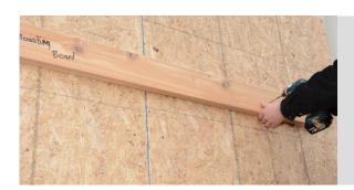
3 Align mark with top of mounting board. Fasten to wall with hardware (not included in kit.)
