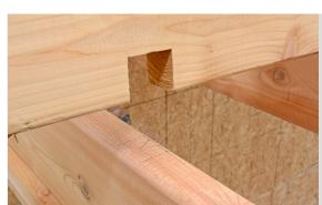
18 Align each of the top runners over the markings on the main runners. It is best to work from one side of the pergola to the next to make sure any bows in the runners are worked out. Attach the top runners into the main runners using 3.5" screws from the top through the pre-drilled holes, until all the top runners are in place.
