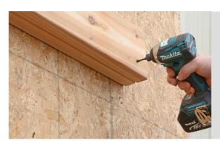
Fasten ledger board to mounting board with 2 2.5" screws every 16 inches.
