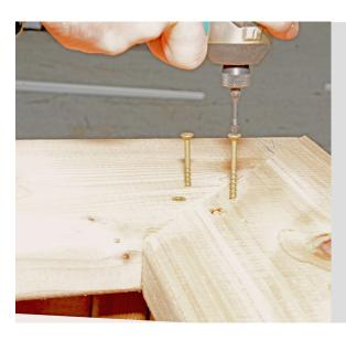
Fasten top plate to posts at corners with 4 3.5" screws.
