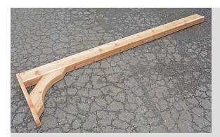
7 Fasten header beam to ledger and mounting boards with 2 3.5" screws.
