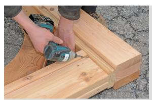
Fasten header beam to post with 5 2.5" screws on each side of beam. Once completed, put in place, measuring from the wall out should be the size of your pergola.
