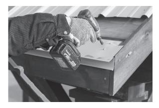
1. The first step will be to install the drip edge. You have to cut these to length. Fasten with one 1" screw. If you have staples or nails, that would be the proper way to fasten. Fasten one every 16".
