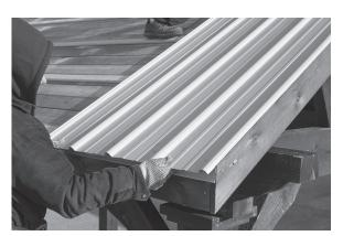
3. Installing the tin starting at one end. There will be an overlap and underlap on the tin. The underlap will have a small flange on. Always start with the overlap on the end of pavilion. Keep the bottom of tin flush with drip edge. Fasten with the 1" screws. You do not have to fasten way on the outside because the gable rake will hold that down. The first piece will have three screws at every lath. Make sure the first piece gets put on square or there will be a problem.
