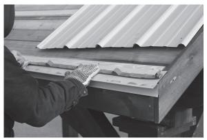
2. Once you have all drip edges fastened, put the rubber enclosure on. Keep it up about 1½" to 2" from bottom of drip edge. This will just paste on. Do not stretch it too hard. The ribs have to line up with the rib of tin.
