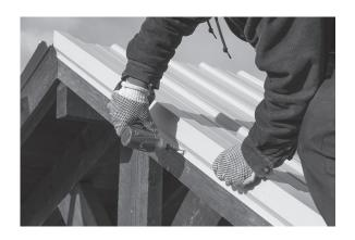
5. Once you have all tin installed, fasten the gable trim. These you have to the angles on the top. Fasten with one 1" screw into fascia and one 1" screw into every lath on other side.
