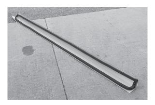
7. When you have all four pieces of rake installed, put the ridge cap on this. You will want to put closure foam on before installing. Peel the plastic off the back then it will just stick to cap.
