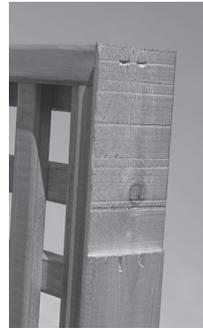
4. Lattice going under 2x6 runner, there will be a notch on one side. Put that side against post.
