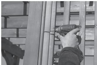
5. Fasten wall to post with three 2½" screws. Once one wall is installed, put 4x4 post in. Fasten post to lattice wall with three 2½" screws.
