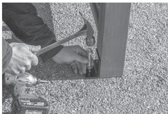
7. Drill a hole with ½" masonry bit going down about ½" farther than length of anchor bolt. Install the wedge anchor the same way you installed the others.
