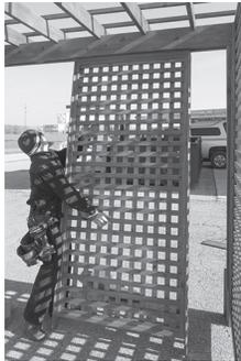
3. Lattice going under header, just push it up between header.
