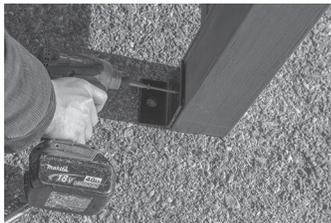
6. Fasten black L bracket to bottom of post with five 2½" screws.
