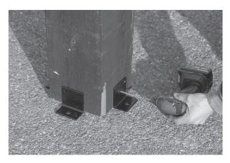
13. Lift bottom post base up approximately 16". You can put a screw in to hold it if you want to. Fasten four of the black L brackets to bottom of post with five  $2\frac{1}{2}$ " screws.
