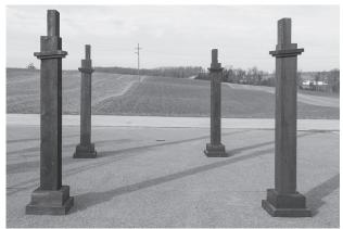
7. The next step is to put the bottom post base and the top trim ring on.
