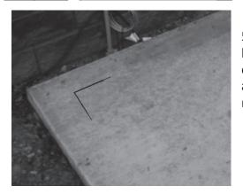
5. Once the template is "square", mark the post locations (using the INSIDE corners of the framed box) on the concrete slab with a pencil. After you have all the post locations marked on the concrete slab, remove and set the wooden template aside.
