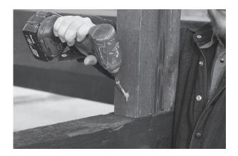
17. You should be ready to assemble the roof structure now. Locate the two pieces about two to three feet long. These go on top of return beam. There should be a mark on top of return beam. Make sure it is right in the center or your rafters won't fit. Fasten it to return beam with two 3½" screws.
