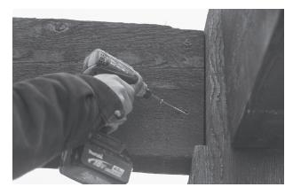
10. Once you have both long headers up, you are now ready to put the return beams in. Make sure the posts are level and at the marks. Fasten the return beams with four  $3\frac{1}{2}$ " screws. Four per side.
