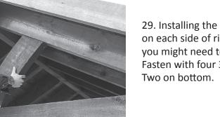
29. Installing the gable decorative trim one on each side of ridge beam support. These you might need to cut down if too long. Fasten with four 3½" screws. Two on top. Two on bottom.
