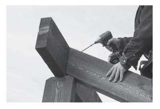
22. The next step will be install the star drive screws. One 5" on top of rafter going into ridge beam. One 8" going into header.
