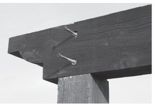
11. You can now go back and put the rest of lag bolts in. These should be the  $\frac{1}{2} \times 9$  lags. Make sure it pulls the return beam in snug against post.
