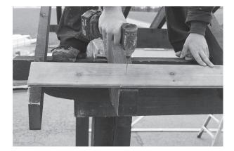
24. The next step will be installing the 1x6 T&G boards. Turn the rough side down. Fasten it with one 2½" screw at every rafter. Continue on up, keeping it flush on both ends.
