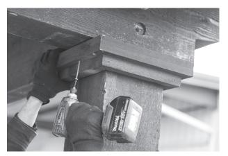
12. The next step will be fastening the top trim to bottom of header with two 3½" screws.
