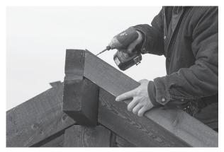
23. There should be four 2x4s the length of rafters. Fasten these to the end of ridge beam with two 3½" screws. Do not fasten the bottom to header.
