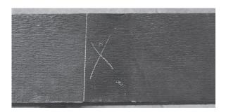
19. Once you have both sides fastened, start on the rafters. Put the four outside ones on first. There will be marks on top of headers. Put the rafters on the X.
