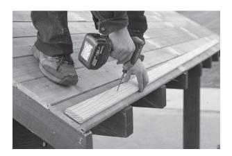
25. Do not do this step if you don't have metal roof. Installing the 1x3 lath, fasten with one 2½" screw. Make sure you fasten where there is a rafter.
