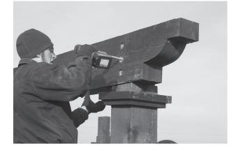
9. Once you have the header beam up in place, fasten it to post with one ½ x 5 lag at each post. Use the center predrilled hole. Do not put the other lags in now. Continue with the other side header.
