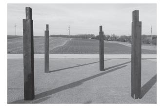
6. The next step is placing the post at the marks you made with the template. When placing the post, make sure you turn it the correct way. There should be a 3" notch and 1" notch on top of post. The 3" notch gets turned to the outside to receive the header beam.
