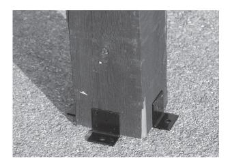
14. When you have all the brackets attached to post, use a ½" mason bit and drill down about ½" farther than length of anchor bolt.
