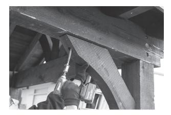
16. The next step will be installing the braces. Fasten brace to header and post with  $\frac{1}{2} \times 6$  lags. There should be a total of eight braces.
