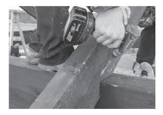
20. Fasten the rafter to ridge beam with one 3½" screw. There is a predrilled hole in rafter. Do not use that now. Fasten rafter to header with four 3½" screws, two on each side. Make sure rafter sits in tight against header.
