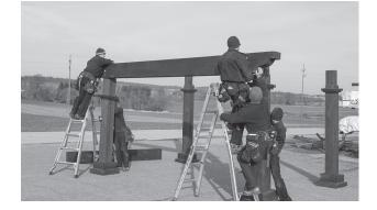
8. You are now ready to install the header beams. If you do not have a couple extra guys to hold the post, you can use the template. Put it together like you did before. Then just screw it to the top of the post to keep the post from falling over.
