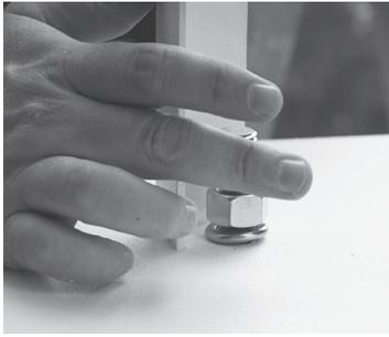
**13.** Tilting the column to one side may make it easier to position the rod so it can be inserted through the hole in the cap. Make sure that the flanges on the plate are oriented properly. Caulk around the center hole. Only finger tighten the stainless steel nut at this time.
