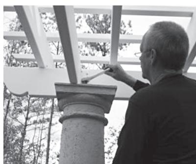
**19.** Set the clutch on the drill to ensure that the screw head does not dimple the top surface of the purlin. Continue across the top of the rafters until all purlins have been installed.
