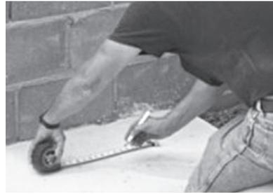
**1.** Locate the center points of the columns. Make sure the layout and slab are square.
