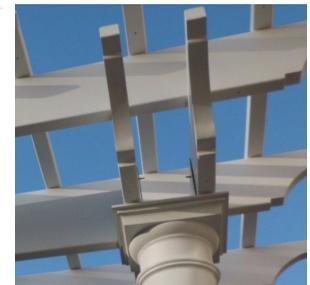
**11-12.** Locate the column cap shown in photos 11 and 12. Place on the column and feed the threaded rod through the hole in the center of the plate with the welded angle.
