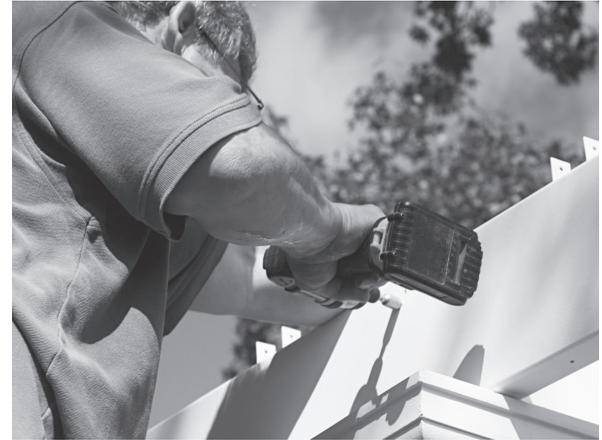
**14.** Install the rafter supports (will have "L" brackets installed to tops of supports) with the decorative rafter tails to the outside of the plate flanges using 2.5" hex head stainless steel self-tapping screws. Set clutch on the drill so the screw is not stripped.
