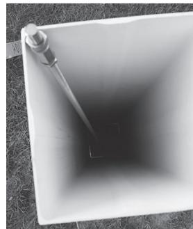
**10.** Screw the threaded rod snugly into the coupling nut at the bottom of the column and tighten with pliers.
