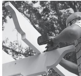
**15.** Starting in the center of the arbor begin installing the rafters with the decorative tails. The rafter supports have fiberglass "L" brackets installed to their tops which indicate the rafter location. **NOTE:** The 1" hex head stainless rafter screws will be used on step # 16 to attach the angle clips to the rafters. (Requires 5/16" socket head bit)
