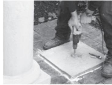
**2.** Use the hammer drill and 5/8" masonry bit to drill a 5" deep hole.
