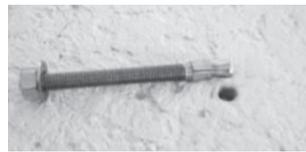
**4.** Use the hammer to install the stainless steel anchor in the prepared hole. **NOTE:** Our 5/8" concrete wedge anchor will install in the prepared hole.
