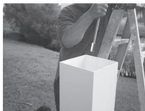
**9.** Lower the threaded rod into the column and engage the coupling nut on the bottom.
