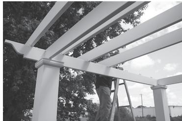
**16.** Starting in the center of the arbor begin installing the rafters with the decorative tails. The rafter supports have fiberglass angles as shown which indicate the rafter location. **NOTE:** The 3/4" hex head stainless rafter screws will be used on step # 16 to attach the angle clips to the rafters. (Requires 5/16" socket head bit) \*Pre-drilling not required.
