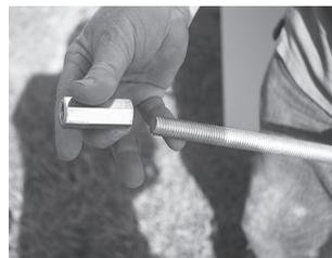
**8.** Attach a connector nut to the threaded rods and then attach the 3" inch stainless steel threaded section to the top of the connector nut.
