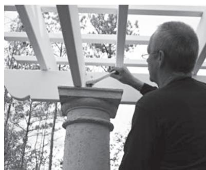
**19.** Set the clutch on the drill to ensure that the screw head does not dimple the top surface of the purlin. Continue across the top of the rafters until all purlins have been installed.
