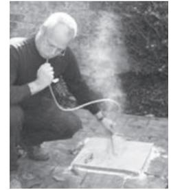
**3.** Remove the dust from the hole to ensure a clear insertion of the stainless steel anchor.
