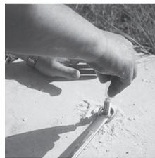
**6.** Install the connector nut on top of the stainless steel anchor and tighten. Use the 13/16" wrench.
