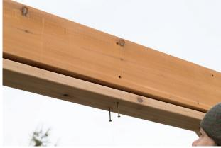
16. Fasten rail to bottom of the header with two2½" screws approximately every 16". Do that with all four sides.
