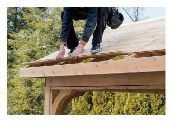
38. Now you are ready to fasten rafter to plate. First take your bottom 1x6 T-G board off. There should be about two or three screws you need to back out. Make sure your ridge beam does not sag in the center. You might need to put a prop in.
