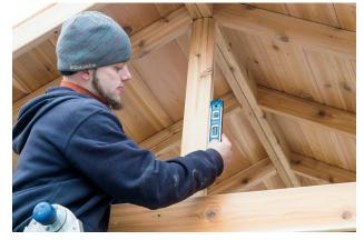
33. Once all the rafters are connected, install the gable sunburst design. Make sure it is in the center of the building. Fasten with four 2½" screws. Two on top, two on bottom.
