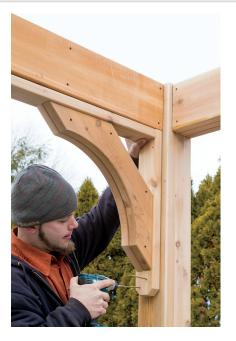
15. Push rail up against the bottom of the header. Put in center of post. Fasten to post with four 2½" screws on both sides. Make sure the screws on the braces are turned in toward the inside of the building.
