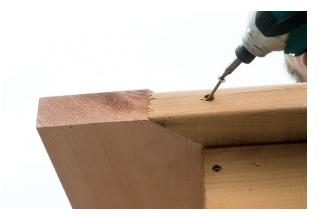
24. Another option is to set all of the top plates into place and put a screw in each corner, then make sure they all line up evenly. Then go back and screw it securely into place every 16" along the top of the header with 2½" screws. Also, drive two 3½" screws from each end of the top plates down into the posts. There will be four 3½" screws per post.
