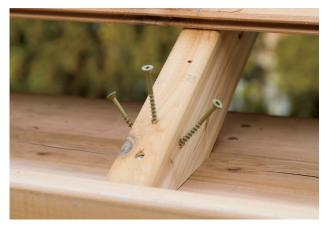
39. Once you have all the bottom T-G off, screw each rafter down into plate with one  $2\frac{1}{2}$ " screw down the center and two  $3\frac{1}{2}$ " screws angled on the sides.
