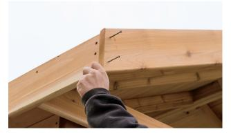
37. Fasten to the 2x4 rafter. One 2½" screw at top and two at the bottom going into fascia. Then one every 16".
