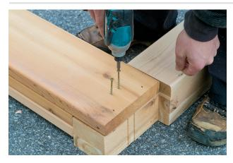
7. Next, assemble two posts and a beam. It is easier to do the longer beams first. Attach beam to post with two  $3\frac{1}{2}$ " screws. You will have some predrilled holes on beam. Do not use those now. Those are for later use.
