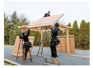
30. Be sure to use a few helpers to get the roofing sections into place. Lift the first section into place making sure the end is resting on the top plate and against the fascia board. The 12" overhang section should be against the inside of the top plate and flush with the outside of the fascia board as shown. Then, use a prop board to hold it into place. (Prop board not included)
