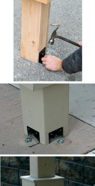
19. Before inserting the bolt make sure that the nut and washer are on, otherwise the bolt will go too deep into the hole. Now insert the wedge anchor bolts into the holes, leaving approximately <sup>1</sup>/<sub>8</sub>" of bolt exposed above the nut. Use a hammer to tap the wedge anchor bolts into the holes.
