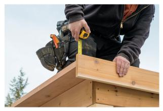
25. Next, install the fascia boards. The fascia will need to sit  $1\frac{1}{2}$ " ( $1\frac{7}{2}$ " with metal roof) up above the top of the top plate boards. It is a good idea to pre-mark these boards. Do so by measuring up  $1\frac{7}{2}$ " on the board and making a mark. Do this toward each inside end of each fascia board, installing the short sides first.
