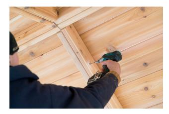
32. Do the same process with the remaining sections until all roofing sections are in place.Once all sections are in place, connect the inside seams of all opposing sections. Do this by driving 2½" screws every 16" along the seams.
