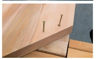
22. Next, install the top plates. These will be two2x12's and two 2x8's. 2x12's go on the long side.They should be about flush on inside of post.Make sure the overhang is same on both ends.Use two 3½" screws to fasten plate to post. Do not cut these without calling.
