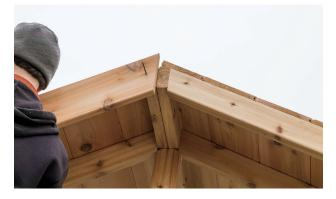
36. Now you are ready to install gable end fascia. These are the boards that have slant cuts on both ends. It might need to be cut down to size. Keep it flush on top of roof panel and center of ridge beam.
