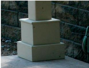
21. When all of the nuts have been tightened down and the posts are securely mounted to the concrete slab, slide the post trim down into place. Next, secure the post trim by using a single 3½" screw, and attaching from the trim into the post.
