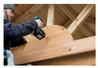
35. Now install the half moon trim pieces. There will be two different sizes. The smaller one goes on top of fascia. The larger one on the inside. These get fastened on all three boards with one  $1\frac{1}{2}$ " screw. Same way with inside one.
