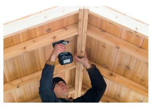
31. Next, set the first roofing section for the other side in place as was done for the first section. These two sections can now rest against each other on their ridge boards. Now, connect these two ridge boards together with 2½" screws, staggered every 16" apart. Make sure the ends of panels are flush.
