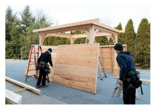
29. When all fascia boards are installed, set the four roof panels on outside of building, you might need 3 or 4 guys for this step.
