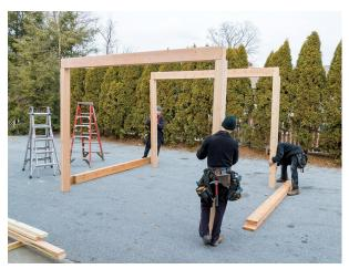
12. Place all posts at the marks you marks you made from template. Get the 2x4 template and screw it to the post. One side to other side to keep it from falling over.
