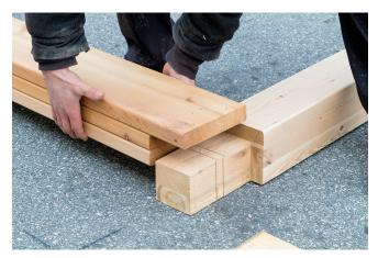
**Note:** Notice that all of the posts will have two sides notched. Turned the notches on the post to the outside to accept the headers.
