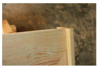
26. Now, hold the first short sided fascia board in place with the mark made resting on the outside edge of the top plate. Also both ends of the fascia board should meet flush with the end of the top plate boards. These you might need to cut down if needed.
