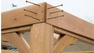
17. There should be 24 pieces of 8" GRK screws in hardware box if you have a standard 4 post structure. Those go at the corners. 6 per corner. Those go in the predrilled holes.
