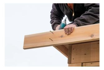
28. The long side fascia boards will overlap the short sides and will extend out past them 11" (12" past the top plate). Notice that they are marked with a line that you will align with the end of the short side fascia board ends. Once in place attach them to the top plate just as was done with the short sides. The long fascia boards will need to be connected to the short fascia boards with 2½" screws. Follow this process until all fascia boards are installed.
