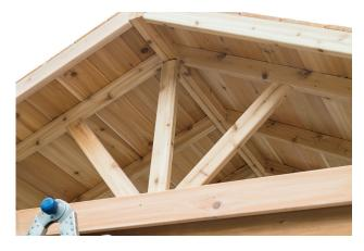
34. Next install the slant pieces. You might have to cut if they do not fit. Fasten with two 2½" screws per board. One top, one bottom.
