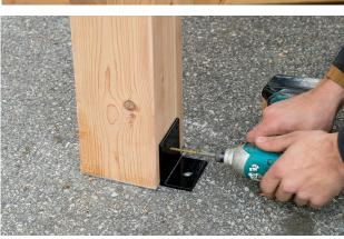
18. Make sure your posts are level and are at the marks on the cement. Fasten the L shaped brackets to post across corner from each other.
