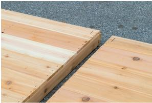
**Note:** The roofing sections will all be marked in the top corner with numbers. Make sure that the roofing sections are set in place so matching numbers rest against each other.
