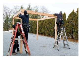
13. Get one of two of your beams and set them in place. Attach with three 3½" screws into other beam. Use the 3 predrilled holes.
