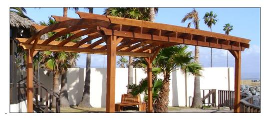
• Option B: With lattice roof. Check you set of drawings and see if right on the center atop the arched rafters there is a roof lattice panel or a slat. You must attach this piece first, and then continue attaching the side panels and slats. Use the deck screws supplied. Attach each roof slat to arched rafters, and attach the roof lattice panels to both roof slats and to the sides of the slats. A screw every 2 or 3 feet is enough.
